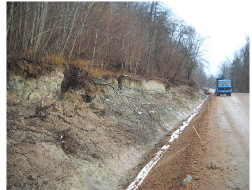
Figure 1. Soil embankment next to the P130 motorway.
