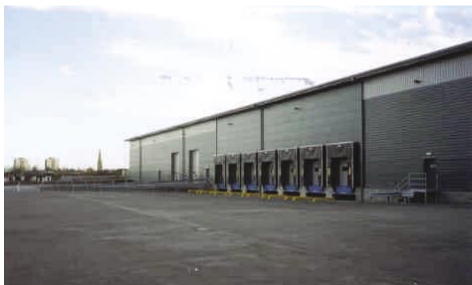
Figure 4: North side of warehouse, Jarrow site
