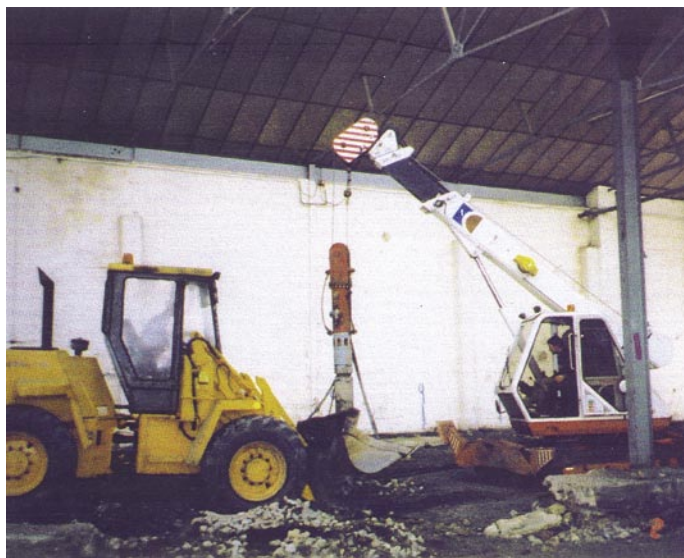
Figure 2: Ground improvement operation, Dagenham site
