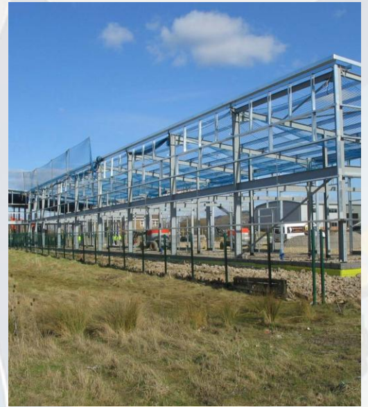
Fig 1, shows construction of phase 2, with the completed phase 1 in the background.
